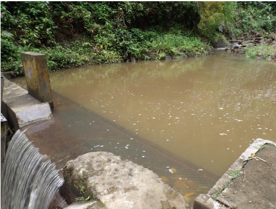
Figure 9.12: Mt. Reuil Dam (2019)
