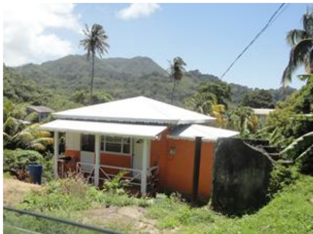
Figure 7.14: Houses in Florida, the community closest to Site F, are provided with electricity and water services
