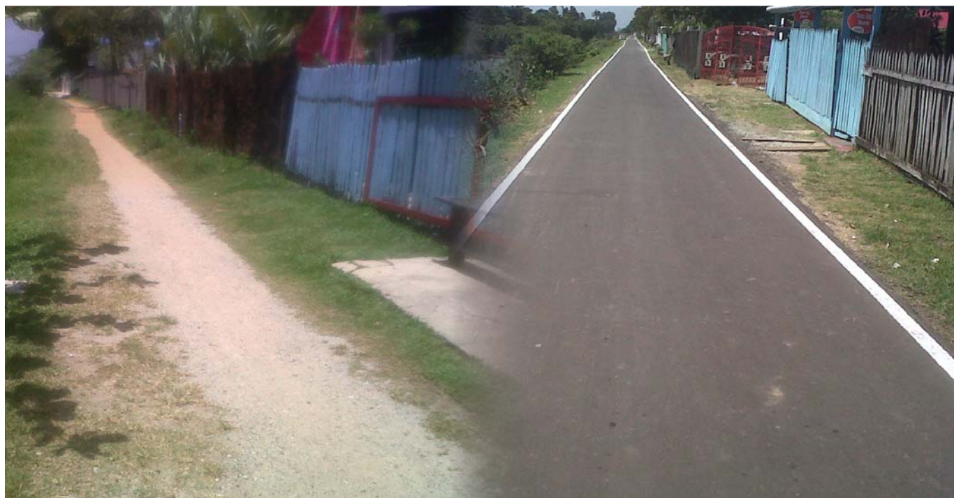
After decades as mostly unsatisfactory pedestrian/cycling dirt tracks the Sideline Dam, Utivlugt, Guyana is transformed into an all-weather road with CDB loan financing.
